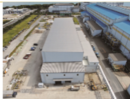
New plant for ultra-fine nickel powder (Wakamatsu Plant)
