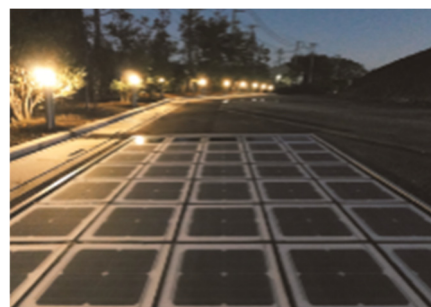
Solar power generation pavement “e-Smart ROAD”
