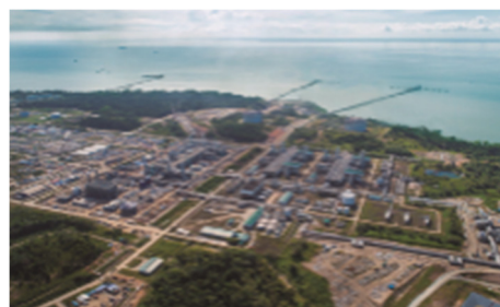
Natural gas liquefaction facilities for the Tangguh LNG Project (Indonesia)
