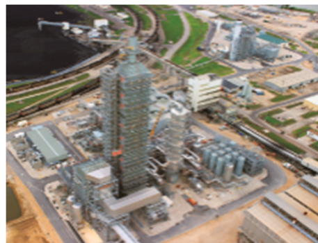
Facilities of the Petra Nova CCUS Project (U.S.)
